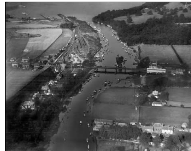
River Leven & Balloch Bridge looking north, 1927 Copyright HES www.trove.scot/image/1256155
